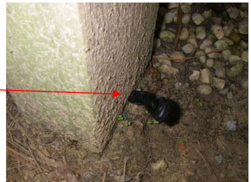
Rot in chase supporting deck Rotten support column (engineer's knife shown)
