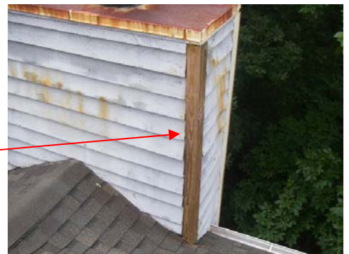
Samples of Chase conditions: Rot Replaced wood, not painted
