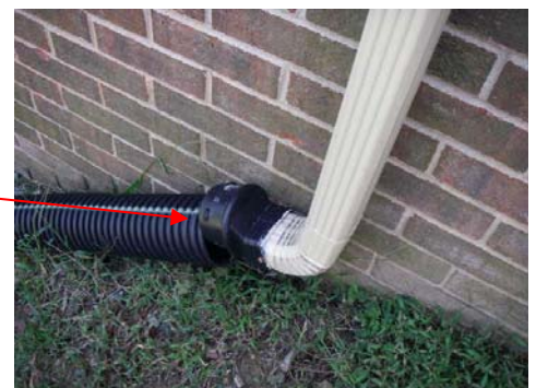
Loose gutter Poor downspout to piping connection
