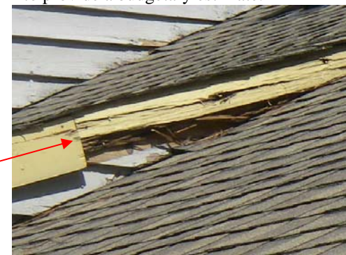
Samples of damaged exterior: Eave end rot Rake trim rot
