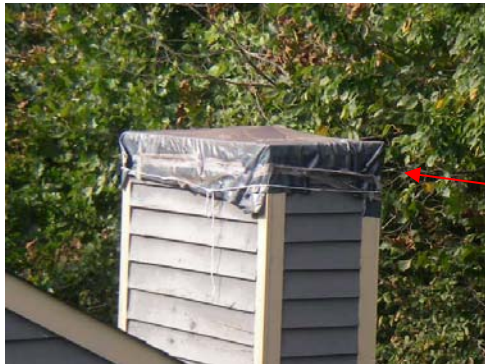
Samples of Chase conditions: Tarp on chase Damaged loose siding
