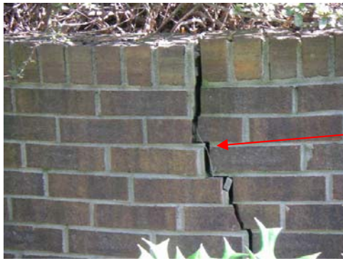
Re-mortar walls
