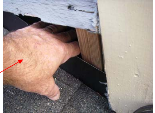
Samples of Chase conditions: Siding rot (engineer's knife shown) Missing siding (hand inside chase)
