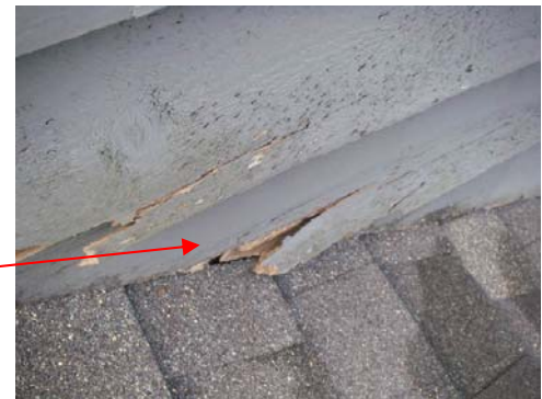
Samples of Chase conditions: Tarp on chase Damaged loose siding
