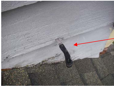
Samples of Chase conditions: Siding rot (engineer's knife shown) Missing siding (hand inside chase)
