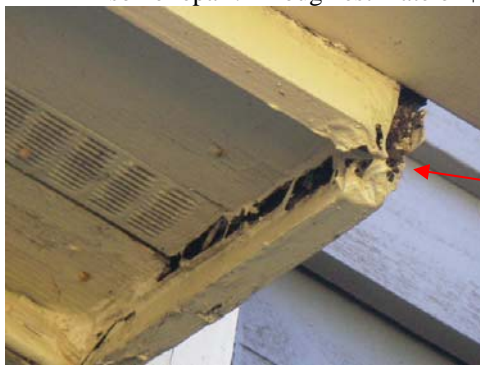
Samples of damaged exterior: Eave end rot Rake trim rot
