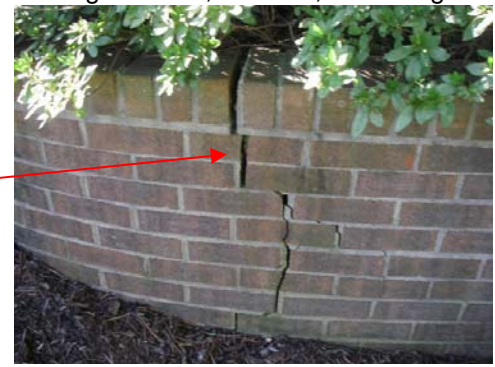
Re-mortar walls
