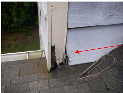
Samples of Chase conditions: Rot Replaced wood, not painted
