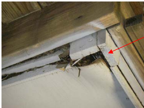
Rot in chase supporting deck Rotten support column (engineer's knife shown)
